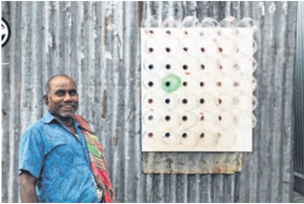
An Eco-Cooler - made of cut plastic bottles mounted on a board with the cut ends facing outside - installed in a window. Hot air entering the bottles is compressed in the bottlenecks, which cools it before it enters the house. PHOTO: GREY GROUP
