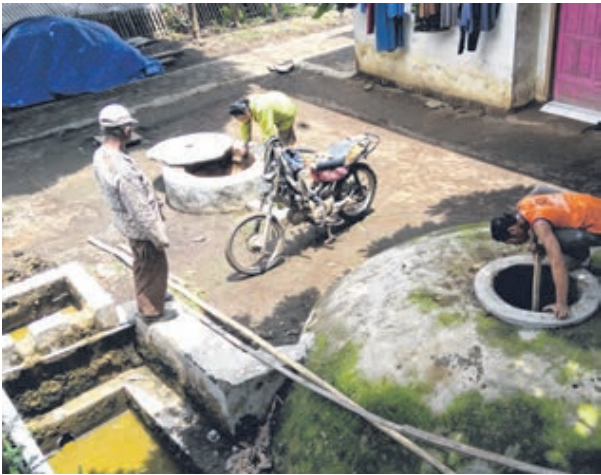
In Kalisari village, tofu makers pipe waste water into containers that generate biogas for homes. PHOTO: KOMPAS
