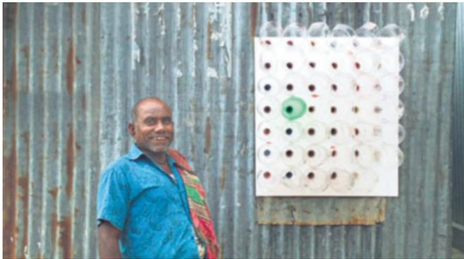
As simple as it gets. The bottleneck principle helps cut temperature as air flows through.
